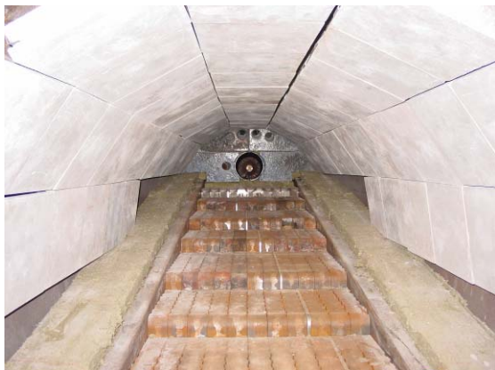
Brennkammer (foto Hollensen Energy A/S)
